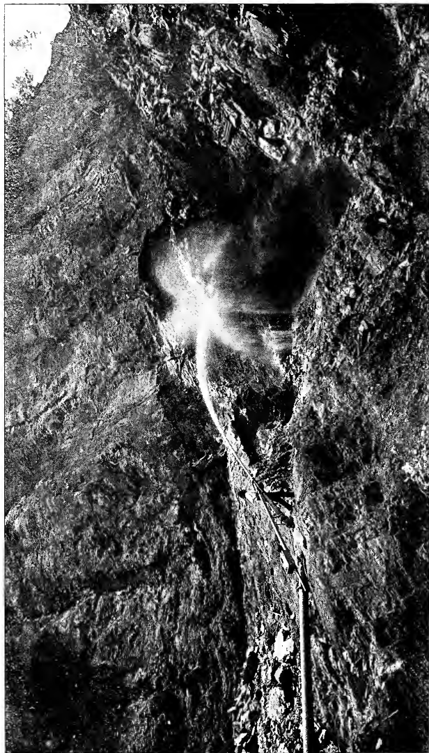
HYDRAULIC MINING AT THE SINGLETON GOLD MINE IN LUMPKIN COUNTY.
