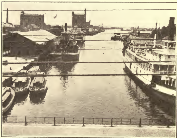
Stockton Channel Looking Down Toward the River
