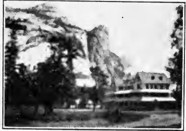
Stoneman House, Later Destroyed by Fire
