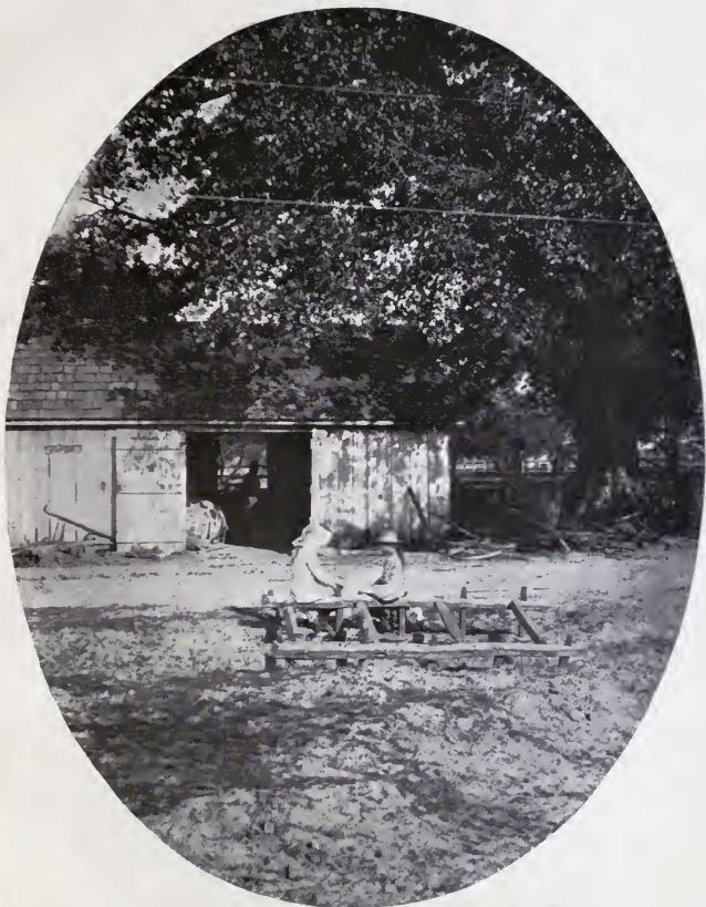
A BAD LIGHTING.
