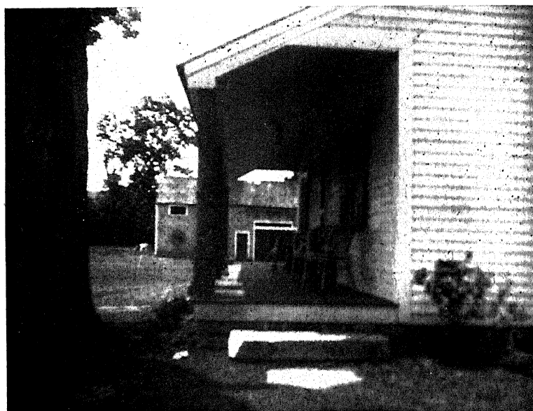
IN RESTORING THE PIAZZA, WE USED SECTIONS OF OLD TELEGRAPH POLES FOR POSTS
