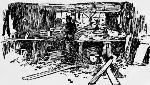
The carpentry shop
