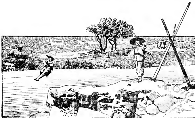
ROPE BRIDGE NEAR TA-CHIEN-LU.
