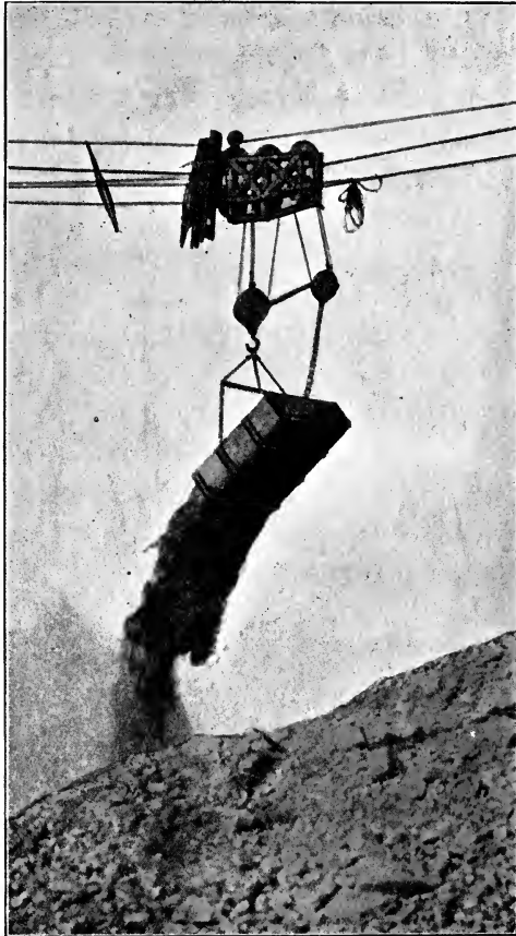
FIG. 139.—Installation for Hoisting and Conveying : Aerial Dump.
