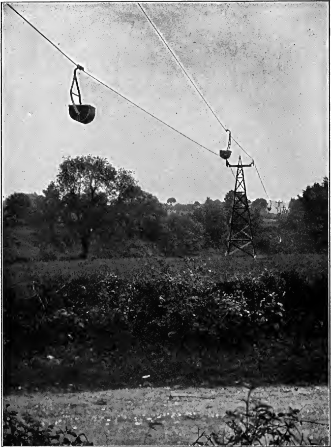
FIG. 99.—Installation at Quarries at Emborough : View along the Line.
