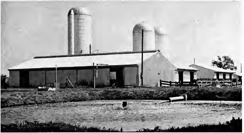
Mechanically aerated lagoon with the dairy housing in the background. (Fig. 23)
