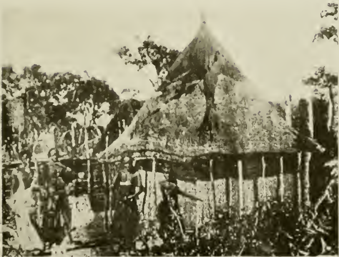
Interior of Valovale Village
