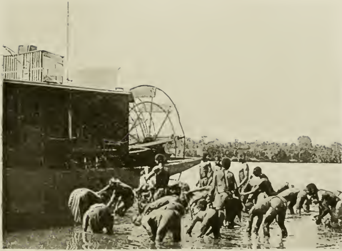
Digging Out the "Centipede"
