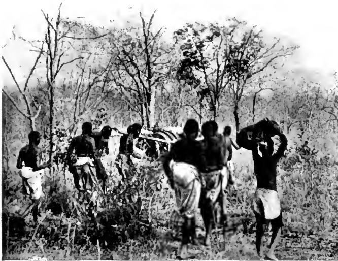
Carrying the Boilers to Chicoca
