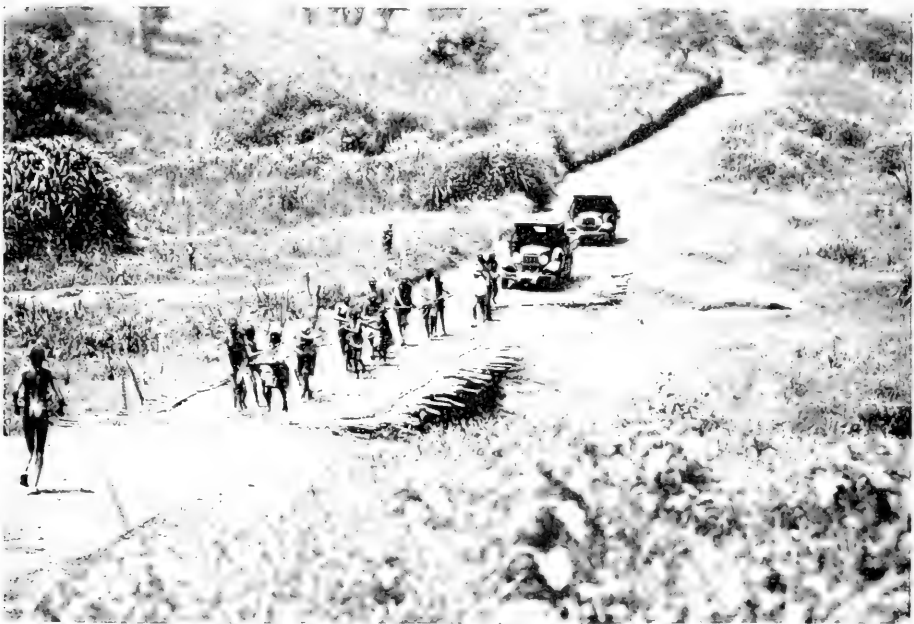
Pulling the trucks over bamboo-covered culverts. The road looks smooth, but it was fresh earth and very soft.
