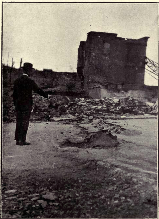
A Crack Across Van Ness Avenue.
