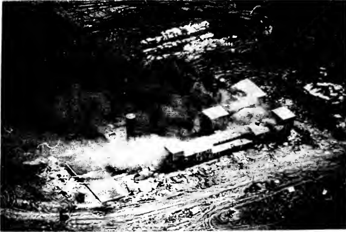
Figure 6. FBI aerial photograph of the Mt. Carmel Center, approximately 6 minutes after the first fire was detected. Rapid fire spread is observed in the southeast tower (fire #1), the dining room (fire #2), and the chapel/gymnasium (fire #3).
