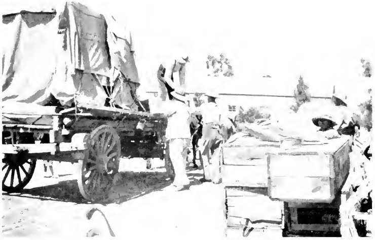
THE ARRIVAL OF REPATRIATION STORES AT A DISTRICT TOWN.
