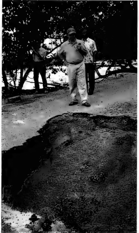
Mahé Island, Seychelles (27 December 2004). President James Michel of the Seychelles inspects damage to infrastructure in the Seychelles. Initial assessments of damage to roads, fishing infrastructure, agriculture, public utilities, schools, land, houses, sports facilities and tourism establishments indicated damage amounting to $30 million. © George Thande/Reuters
