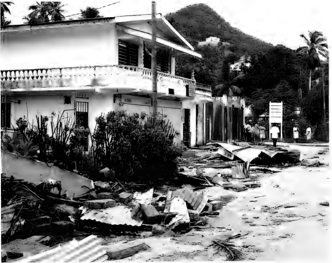
Mahé, Seychelles (26 December 2004). People assess the damage after the tsunami hit the Seychelles capital Mahé. Seawater surges flooded the low lying areas of Mahé, Praslin and La Digue and caused widespread damage to beaches, coastal vegetation, roads, bridges, houses and other infrastructure. The tsunami was followed on 27 December by extreme weather, with rainfall reaching 250 millimetres in the northern and central areas of Mahé. Torrential rains continued for several days, causing further damage to infrastructure, dwellings and vegetation. © Terence Fortune/Reuters
