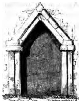
Barnack Church, Northamptonshire.
