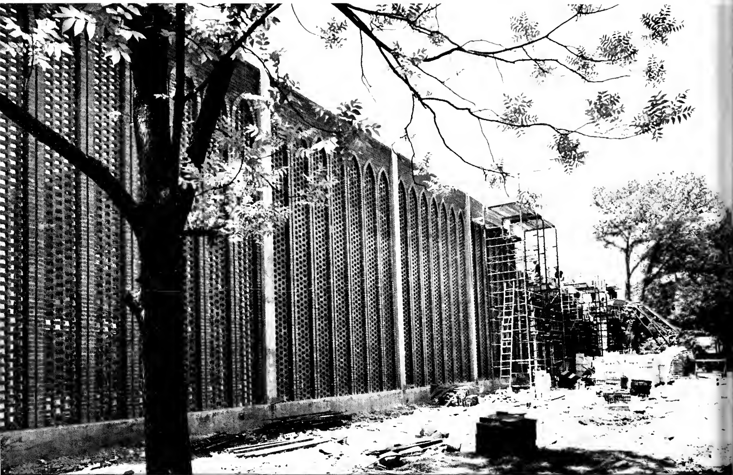
A magnificently tall pierced-brick wall will be the architectural feature of the Dana Fine Arts Building.
