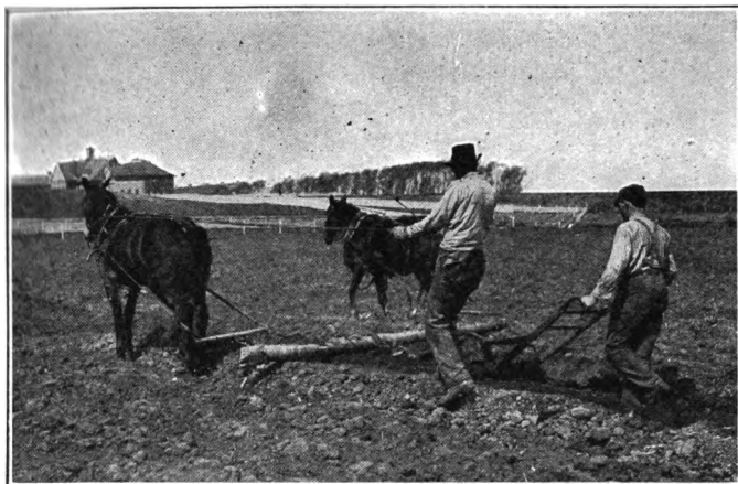
Fig. 61. Filling the ditch with a plow.
