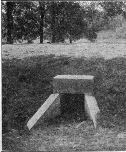
Fig. 97. Concrete culvert after the plan of Fig. 96.
