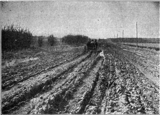
Fig. 81. A typical condition of an earth road on which the drag has not been used.
