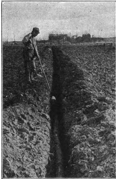
Fig. 59. Laying tile with the tile hook.
