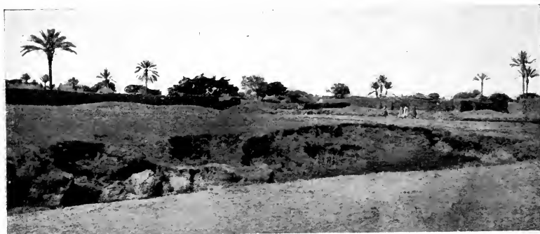
NEAR THE SOUTHERN GATE, ZARIA.
