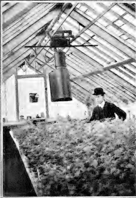
Thwaite Electro-Culture System - Rear Side of the Arc Light. From The Scientific American .
