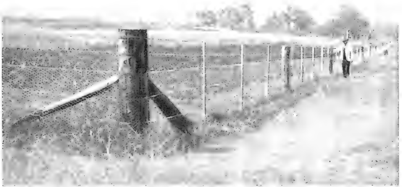
A wire-netted rabbit-proof fence, two posts and six droppers per chain.
