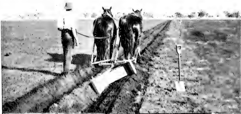
Home-made crowder at work making the channels; a valuable implement.
