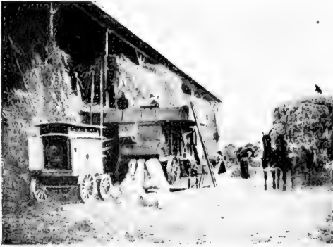
Portable Motor attached to Threshing Machine on a German farm.—Illustration by Siemens Bros., Ltd.
