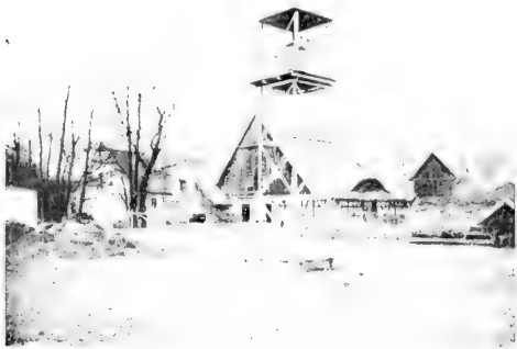
Stationary Transformer on a German farm, connected with a supply station. From this point the current is transmitted all over the farm.—From illustration kindly lent by Siemens Bros., Ltd.
