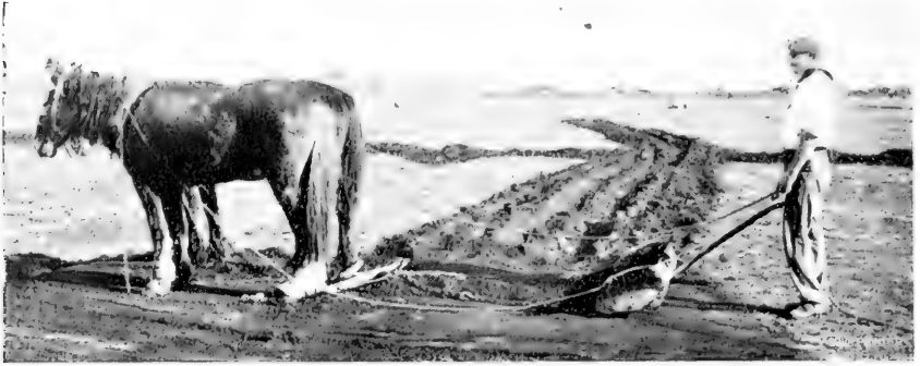
Contractor working buck-scraper.
