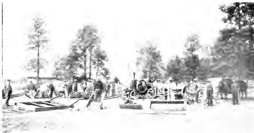
Workmen who have been employed in laying out and planting the orchard, and putting in crops, fencing, &c., and carpenters who have put up the buildings, together with implements used on the station.
