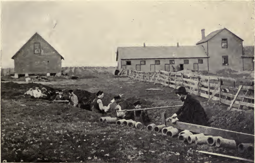
FIG. 27.—Class of boys laying a tile drain, as illustrating work under an instructor on a school farm or on a neighboring farm.
