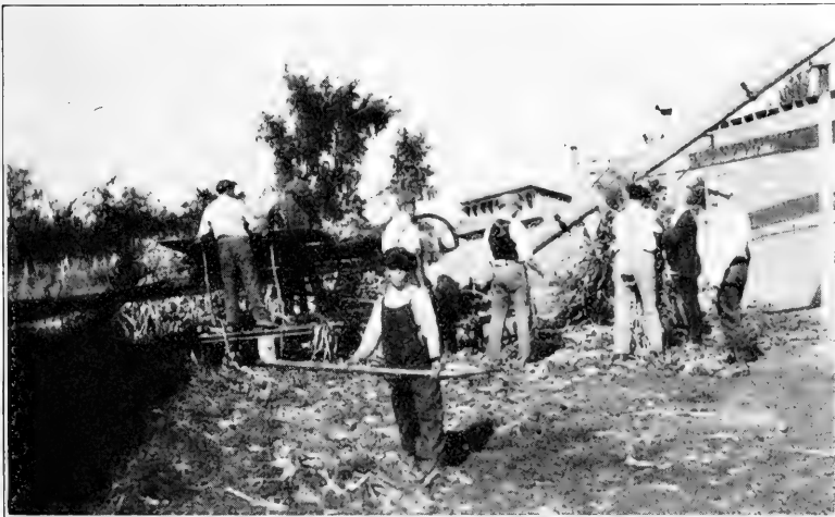
FILLING THE SCHOOL SILO AT WEST SIDE, GREEN BAY HIGH SCHOOL.
