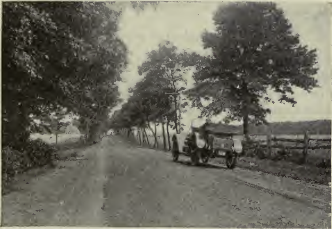
Bituminous macadam road in New Jersey.
