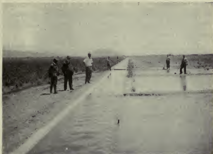
Flooding from cement ditches.
