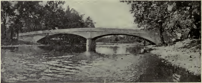
A concrete bridge. This type of structure should replace the old wooden bridge.
