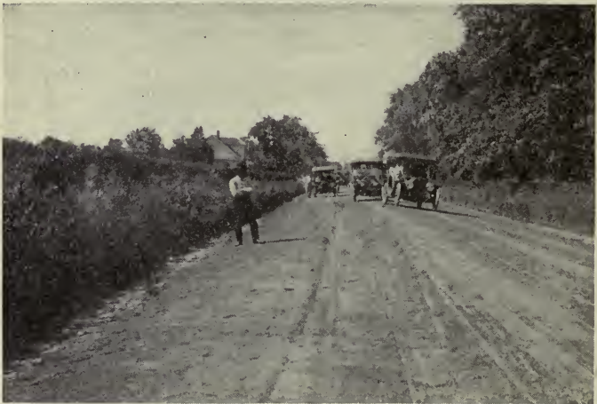
Earth road in Kansas.
