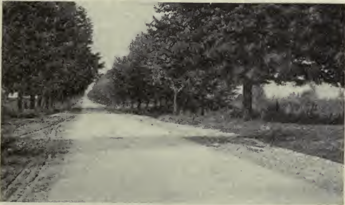
Concrete road near Detroit.
