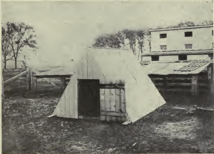
Individual hog cot, on rumers, so that it can be drawn from place to place.
