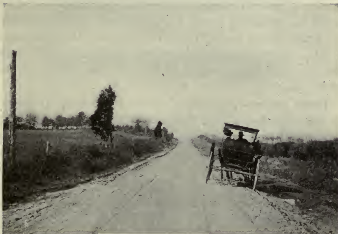
The same road improved.
