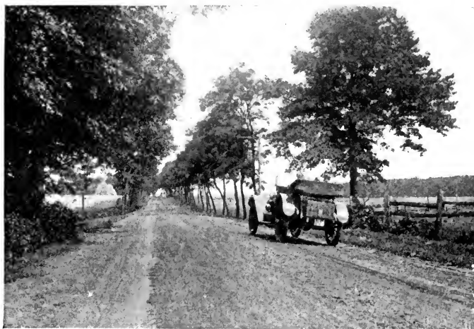
Bituminous macadam road in New Jersey.
