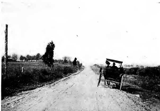
The same road improved.
