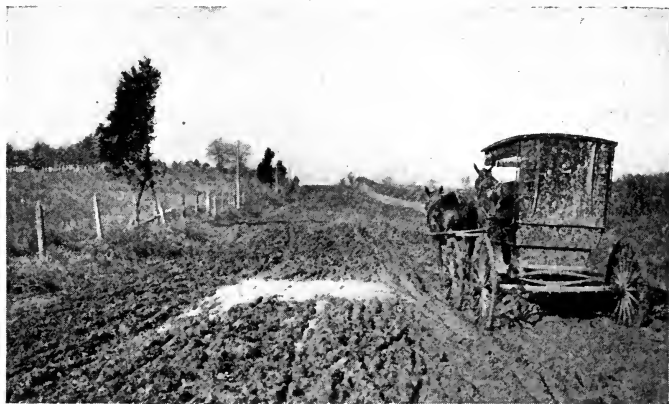
An earth road that needs improving.
