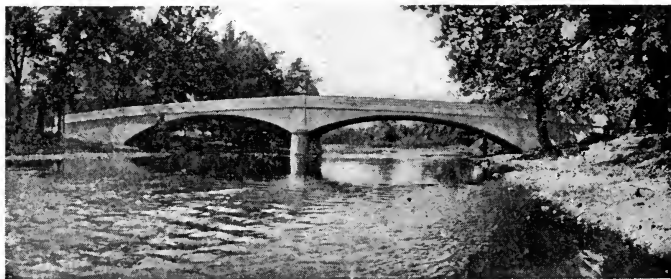
A concrete bridge. This type of structure should replace the old wooden bridge.
