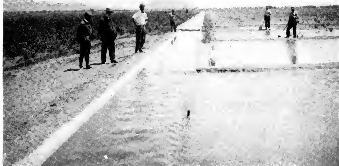
Flooding from cement ditches.
