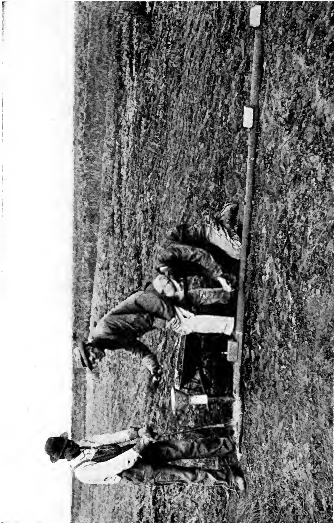
Sub-irrigating method. Continuous piping system.
