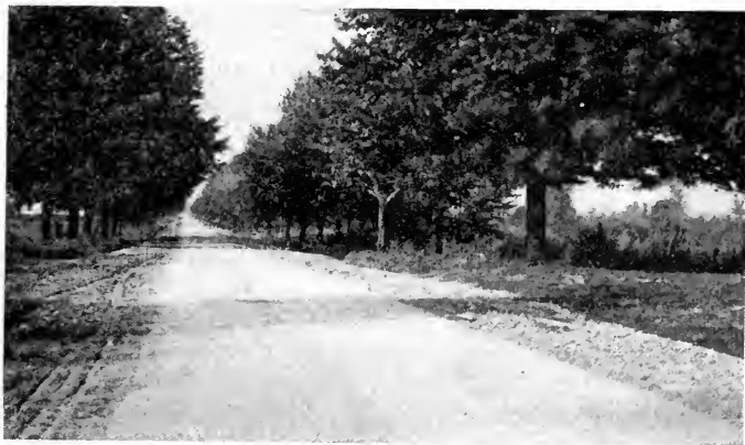
Concrete road near Detroit.
