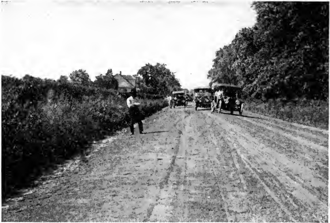
Earth road in Kansas.
