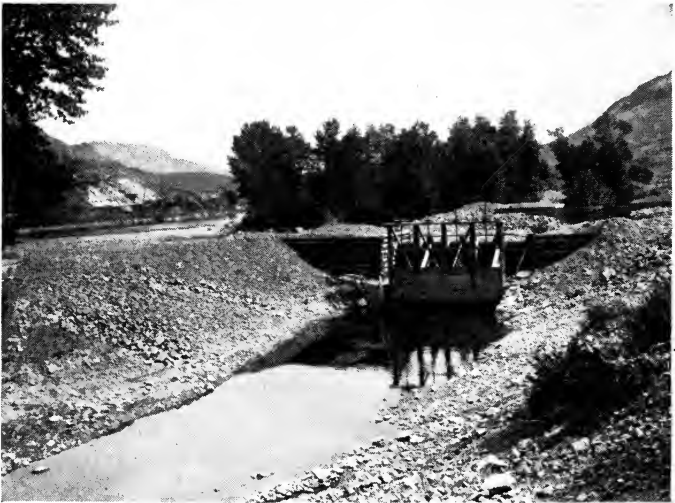
Regulating gates and inverted siphon. Chestnut Valley, Missouri River, Montana.
