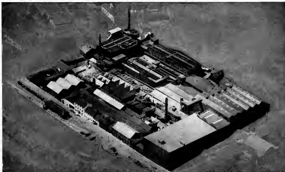
ONE OF OUR WORKS AT PORT DUNDAS, GLASGOW.
