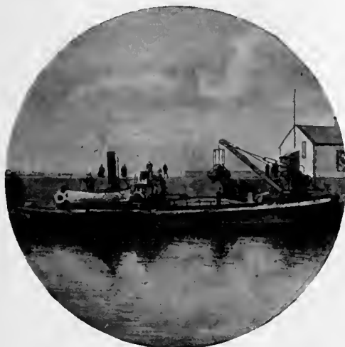
"KINGSTON" DREDGER, on Barge. Drague "Kingston," sur chaland. Draga "Kingston," instalada en una barcaza.
