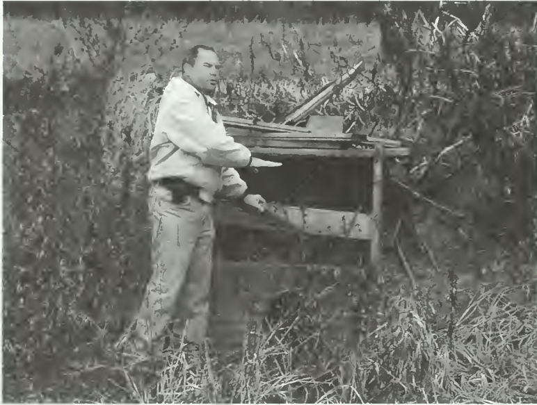
Boards placed in stop log flood control structures are used to control water depth in flooded fields to enhance waterfowl habitat.
