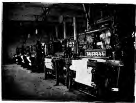
INTERIOR VIEWS OF TEXTILE BUILDING.
