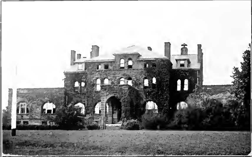
HOLLADAY HALL, ADMINISTRATION BUILDING
