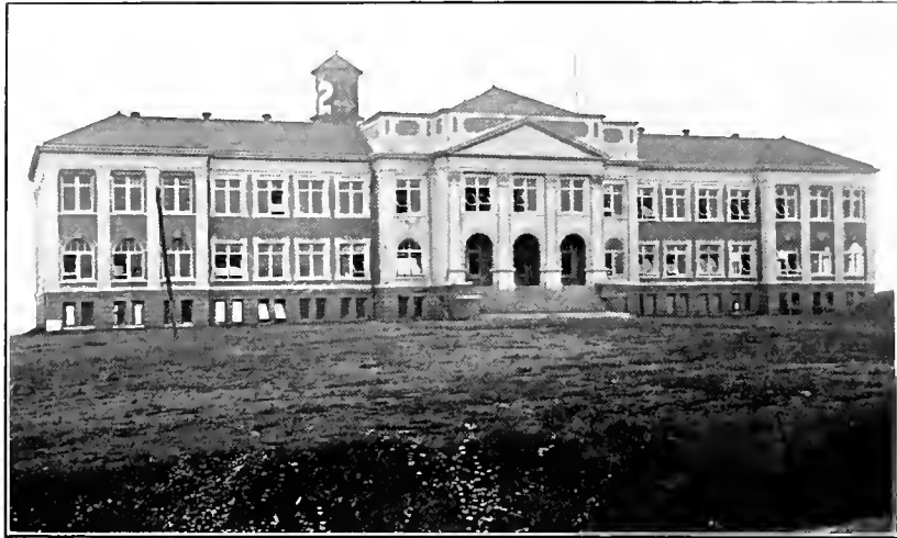
PATERSON HALL, AGRICULTURAL BUILDING
