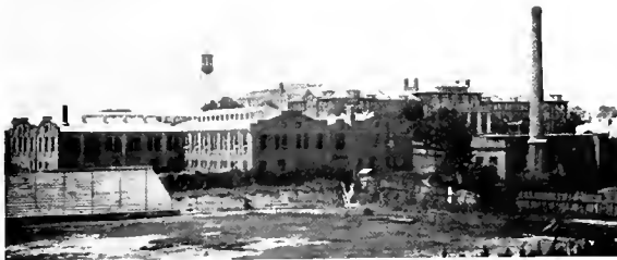
POWER HOUSE AND SHOPS
