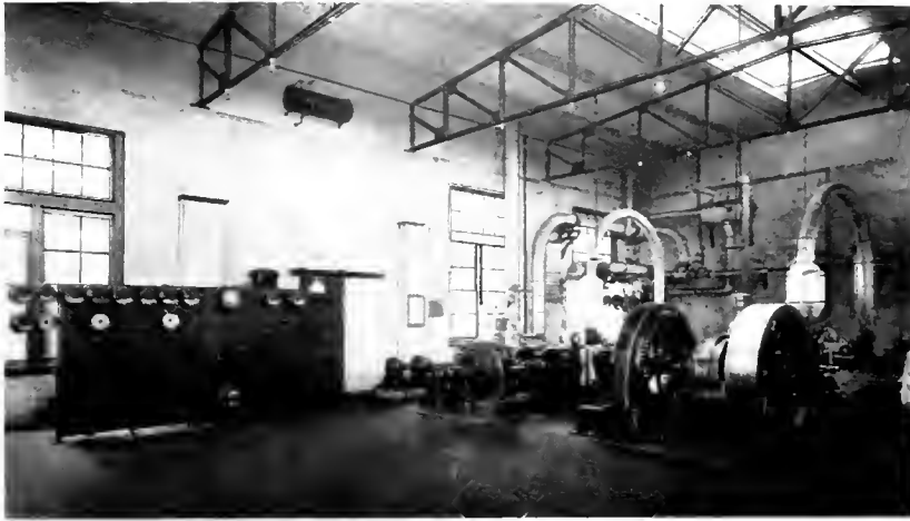
COLLEGE POWER PLANT
