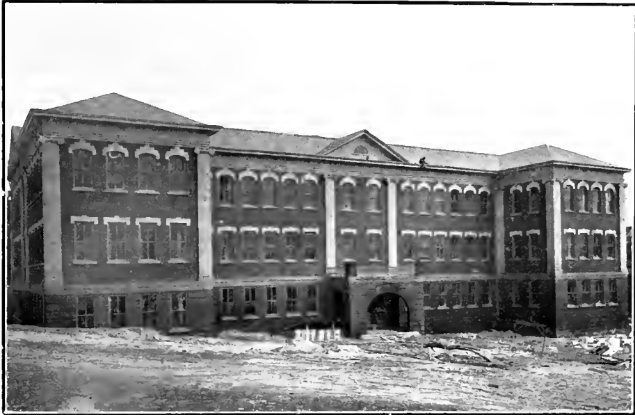
CIVIL ENGINEERING BUILDING (REAR)
