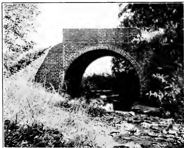
BRIDGE ON COLLEGE FARM
