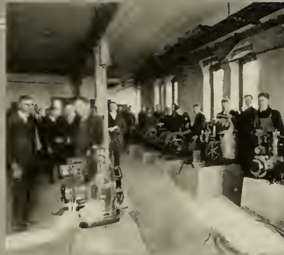
GAS ENGINE LAB.
