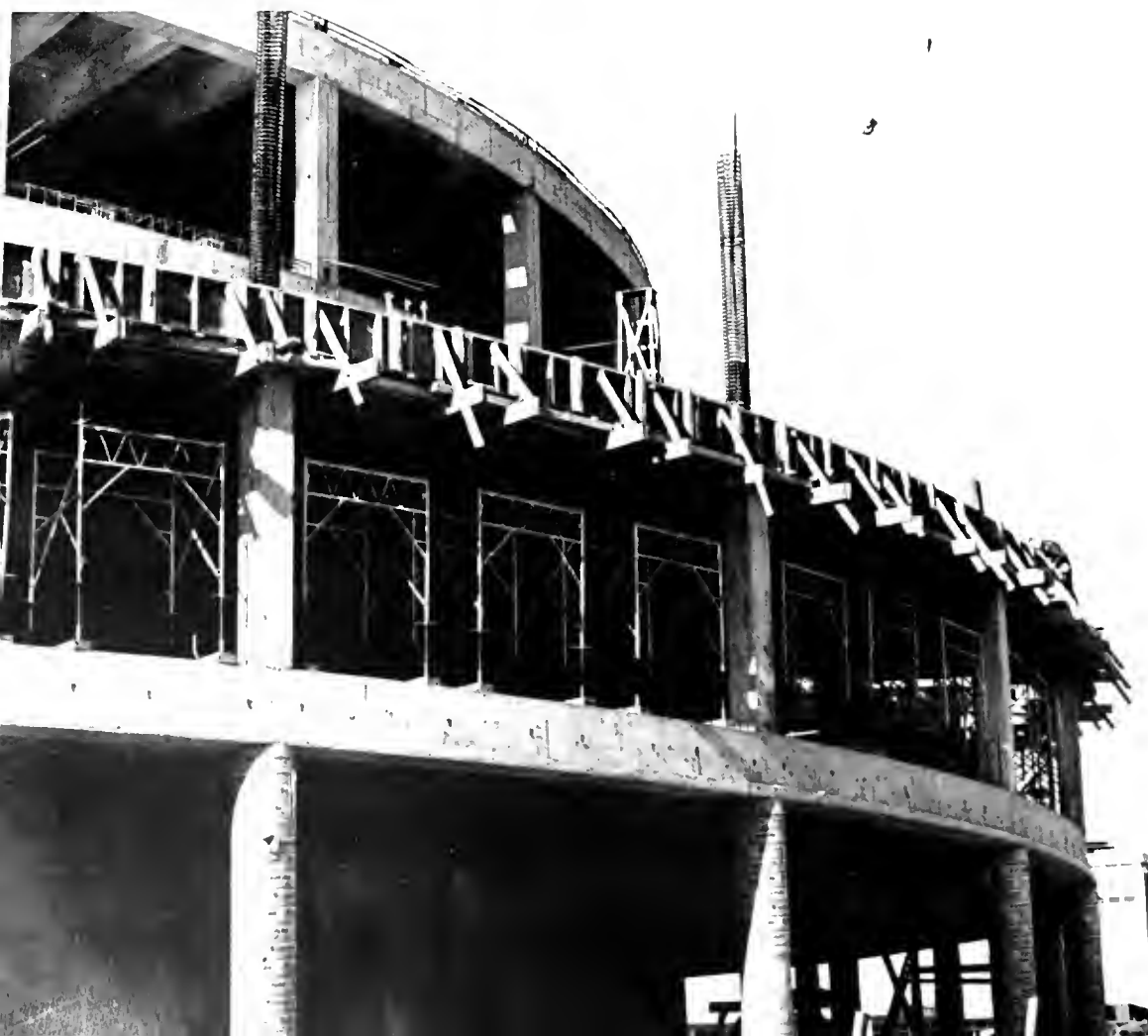
Circular classroom building will be completed next fall. . . .
