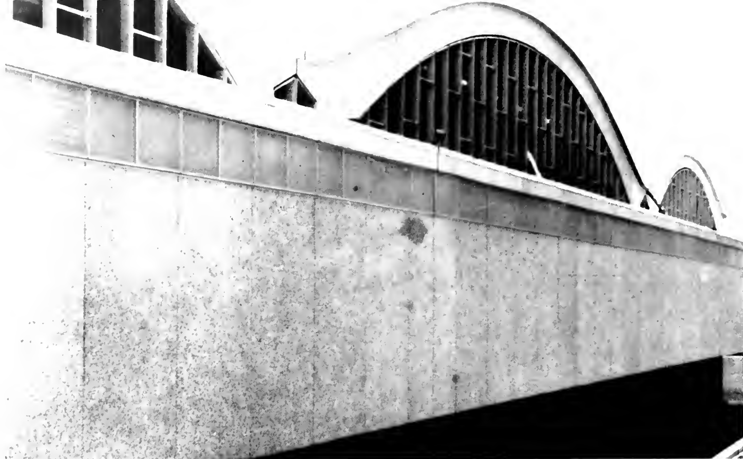
Modern architectural influence is evident in the new gym. . . .
