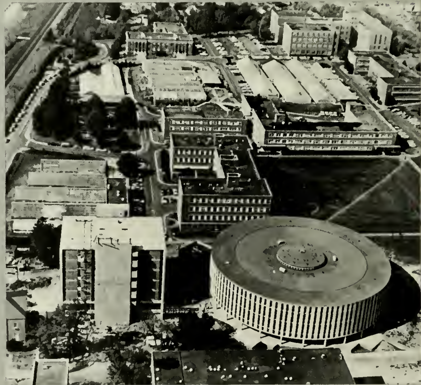
Above: In vicious contrast to Bragaw, the doughnut-shaped Harrelson Hall was built in 1961. There were numerous construction problems, notably the fact that the building sank into the supporting soil, because no one bothered to check what kind of ground the building was being erected upon. There are many students who wish that the building would sink into the depths, simply because most math classes are held in Harrelson.
