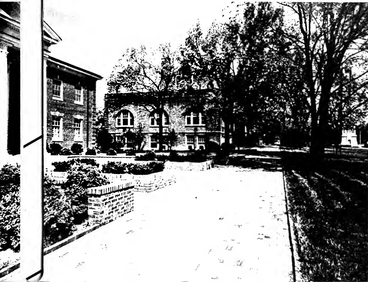
This perspective of the eastern border of campus shows the Alumni Building and gives a glimpse of the Belltower, along Pullen Road.
