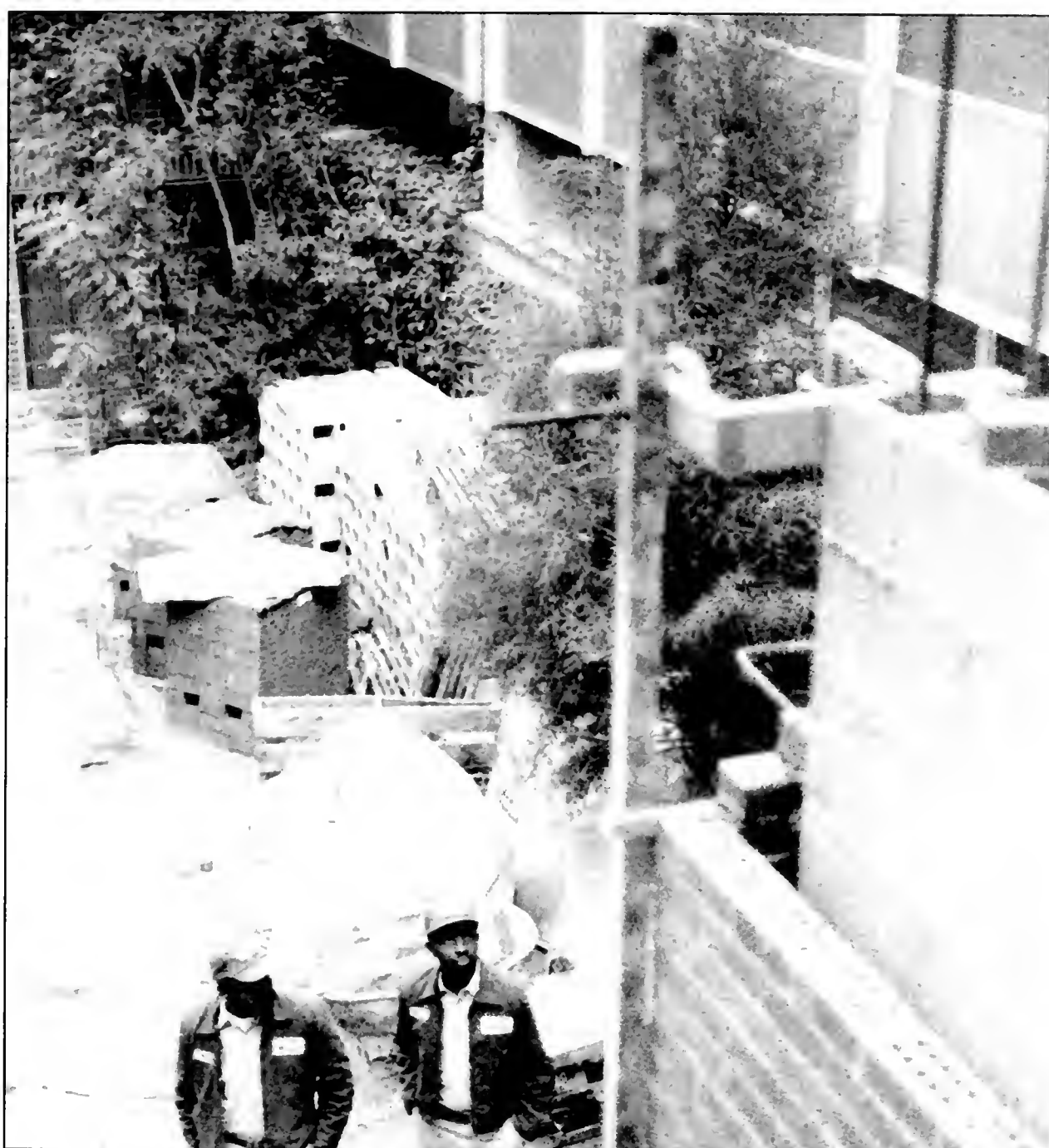
Elevator construction on campus. Photo by Martha Harvey.
