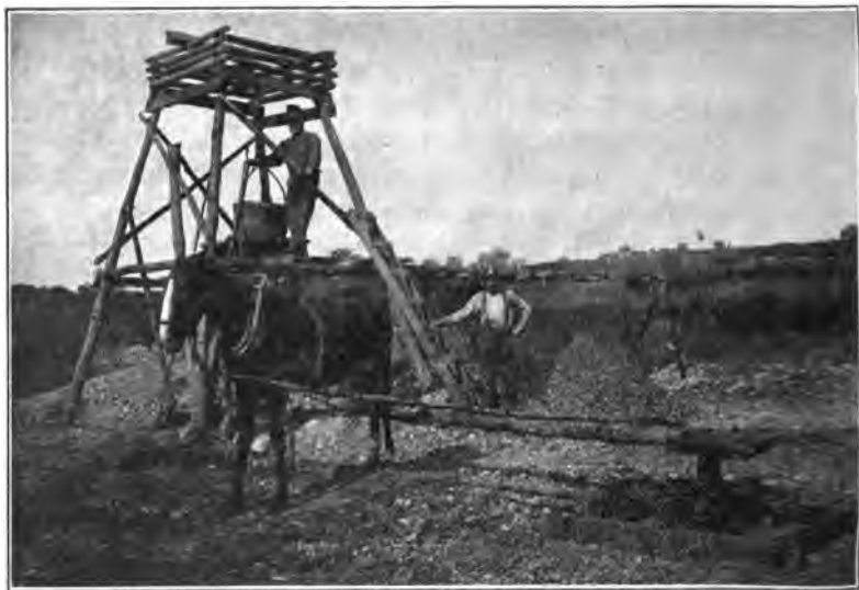
OLD TIME METHOD OF MINING LEAD AND ZINC ORE WITH A HORSE HOISTER
