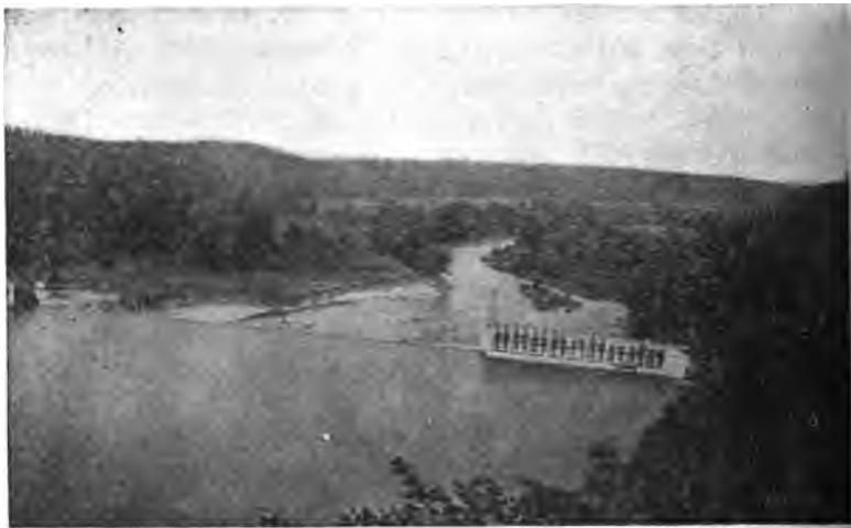
DAM ACROSS WHITE RIVER AT POWERSITE, MO., FORMING LAKE TANEYCOMO
