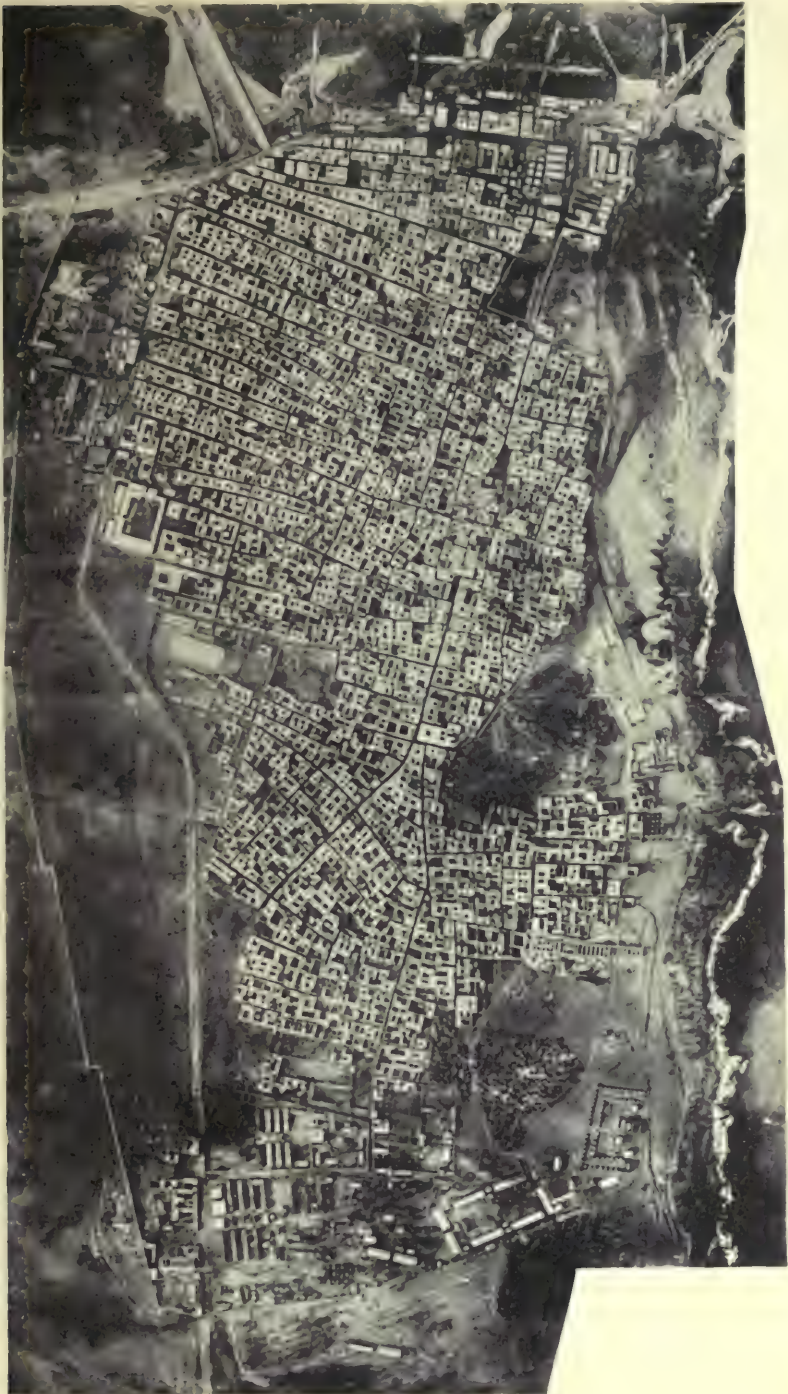
FIG. 207.—Bengasi, a North African town, surveyed for the first time from the air. Italian official photograph.
