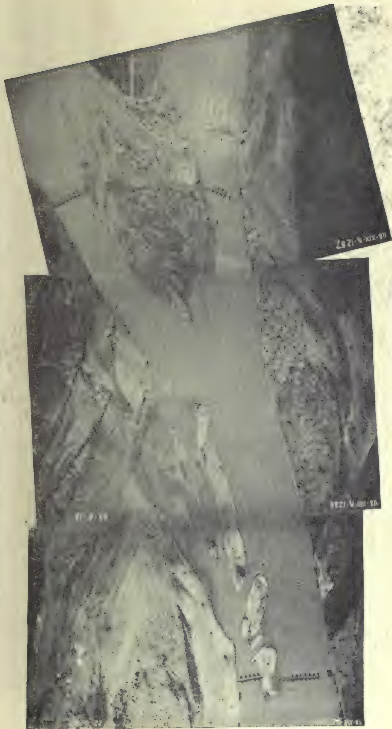
FIG. 124.—The Piave River. To left, destroyed bridge, to right, pontoon bridge under construction. Italian aerial photographic service.
