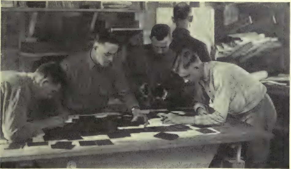
FIG. 141.—Scaling negatives for mosaic map-making.
