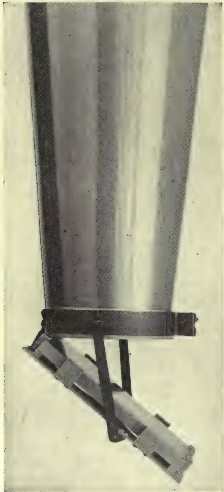
FIG. 148.—Mirror on camera cone for taking oblique views.
