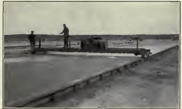
FIGURE 16. "CURING COMPOUND" BEING SPRAYED ONTO FRESHLY LAID CONCRETE PAVING
