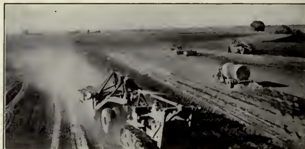
FIGURE 5. LEVELING OPERATION IN FOREGROUND; WATERING TRUCK IN CENTER BRINGING SOIL TO PROPER MOISTURE CONTENT; COMPACTION IN REAR
