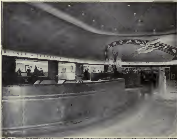
FIGURE 7. LOBBY, NEW YORK AIRLINES TERMINAL
