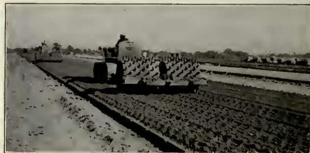
FIGURE 6. CLOSE-UP OF COMPACTION BY MEANS OF SHEEP'S-FOOT ROLLERS
