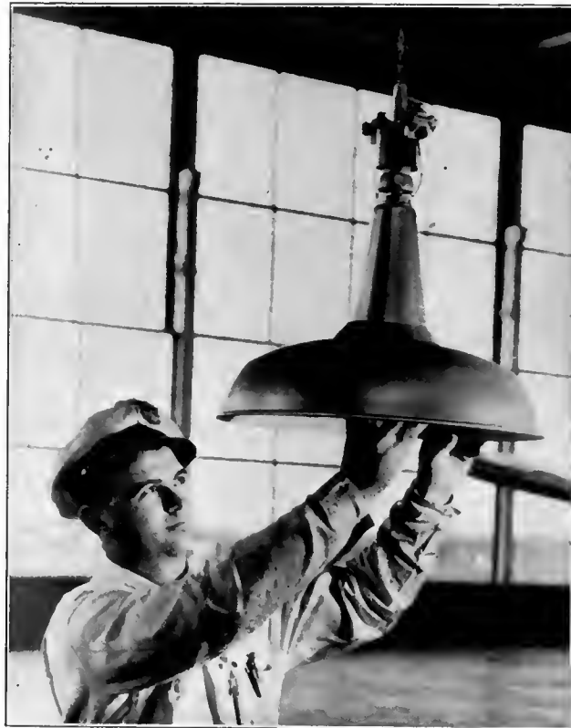
Courtesy Thompson Electric Company Fixture Being Serviced from Floor
