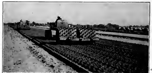
FIGURE 6. CLOSE-UP OF COMPACTION BY MEANS OF SHEEP'S-FOOT ROLLERS
