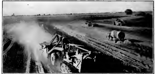
FIGURE 5. LEVELING OPERATION IN FOREGROUND; WATERING TRUCK IN CENTER BRINGING SOIL TO PROPER MOISTURE CONTENT; COMPACTION IN REAR
