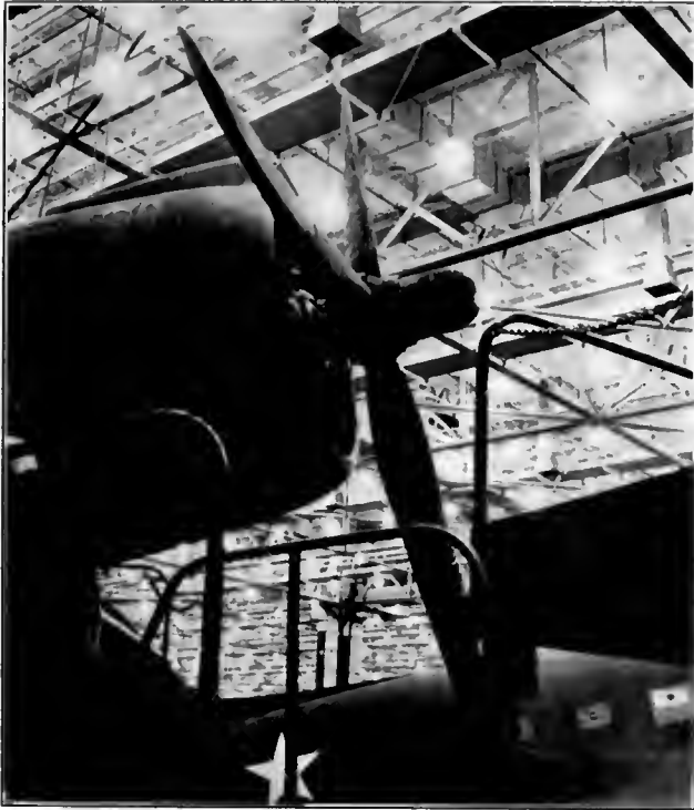
Courtesy Holophane Company, Inc. Catwalks for Servicing Lights
