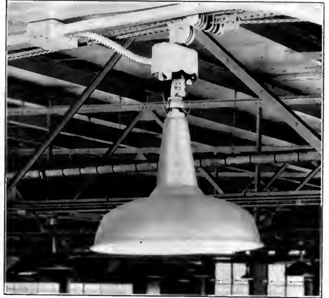
Courtesy Thompson Electric Company Thompson Hangar, Showing Chains for Lowering to Floor
