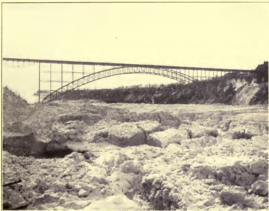
One of the reasons why the auxiliary steam plant is necessary in the light and power industry.
