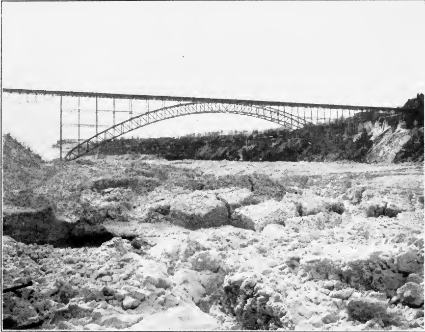
One of the reasons why the auxiliary steam plant is necessary in the light and power industry.
