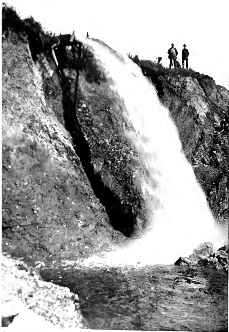
IT IS THE WATER DO THE WORK. GROUND SLUICING ON DANIELS CREEK, NEAR NOME, ALASKA
