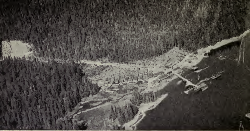
An aerial view of Camp Three, the main camp of the Alaska Spruce Log Program, on Kosciusko Island, Tongass National Forest. The quarry shown at the left produced the rock required for surfacing the logging road. (Courtesy U.S. Forest Service.)
