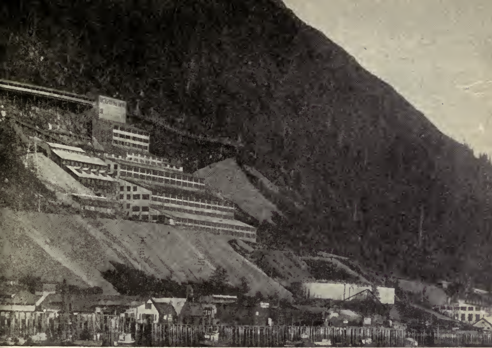
Alaska Juneau gold mine, one of the largest low-grade gold-ore mines in the world. Its unique feature is that the shafts go up instead of down.
