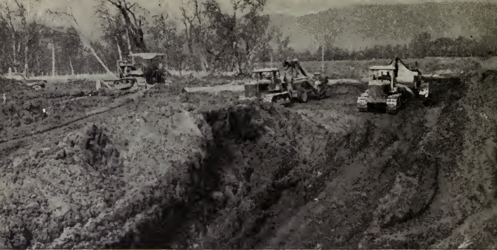
Grading on the Glenn Highway, Mile 3 from Palmer—a relocation of the old road. (Courtesy Alaska Road Commission.)
