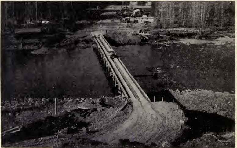
A temporary pontoon bridge spanning a river on the highway is pictured above. The permanent bridge built to replace it is shown below.
