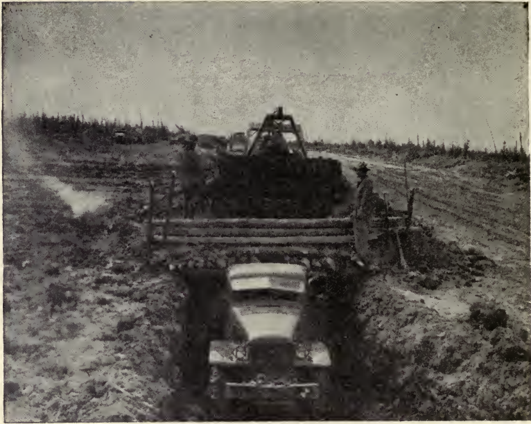
A novel system of loading dirt in the absence of shovels. The truck backs into the depression and is loaded from above by a bulldozer.
