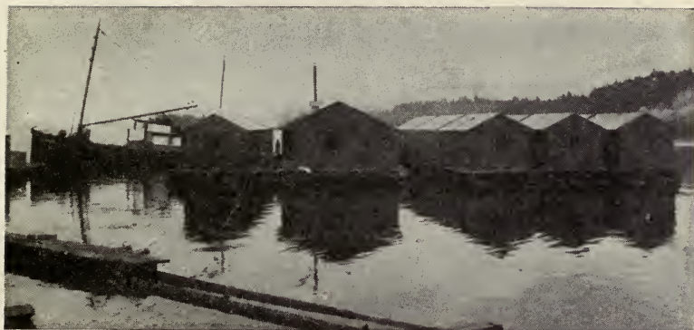
One of the floating camps used by the Alaska Spruce Log Program. As most merchantable timber is located close to tidewater, loggers can be housed in this manner. (Courtesy U.S. Forest Service.)
