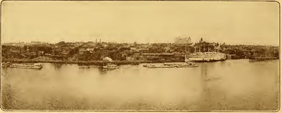
ALBANY FROM ACROSS THE RIVER
