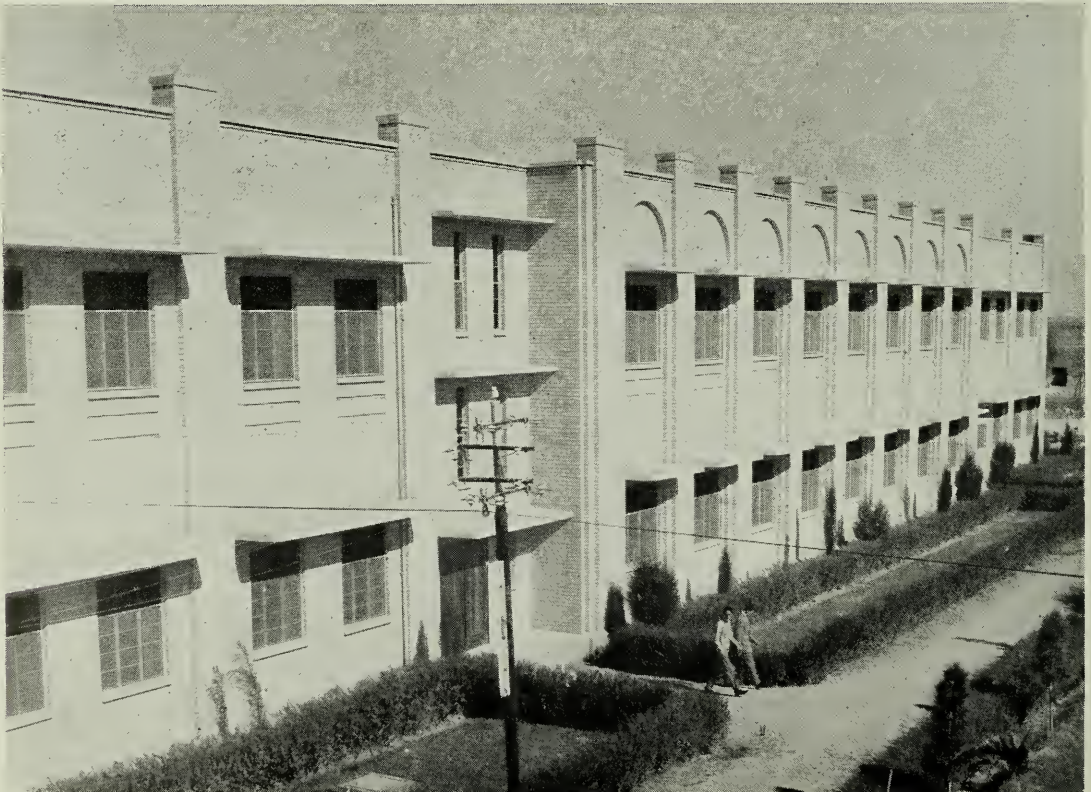
THE BUSINESS BUILDING
