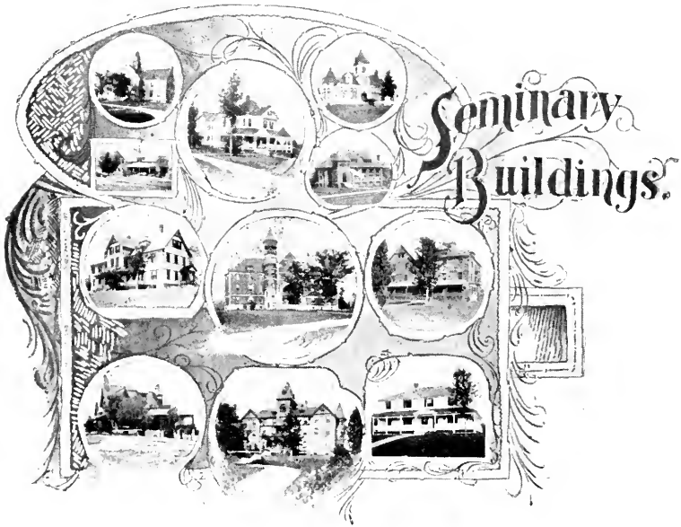
Left row, beginning at top: Stone Hall, Holton Hall, Betsey Moody Cottage, Reveil Hall. Centre row: Moore Hall, Marquand Hall, East Hall. Right row: Talcott Library, Skinner Gymnasium, Weston Hall, Hillside Cottage.
