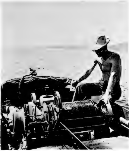
Fig. 8 Winch and cable in dredge boat
