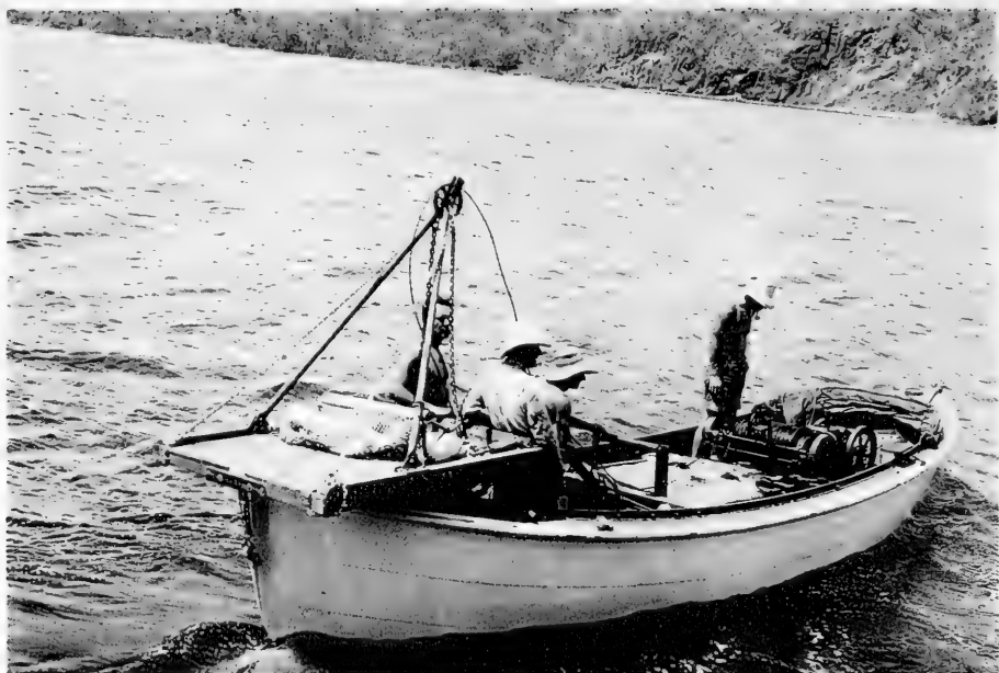
Fig. 11 Old dredge boat
