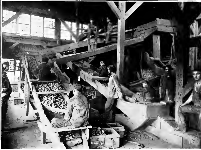
Slate Pickers, Interior View of Breaker
