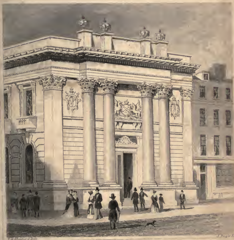
THE NEW GRESHAM COLLEGE LONDON
